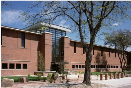
Denver Federal Center Lakewood, CO
